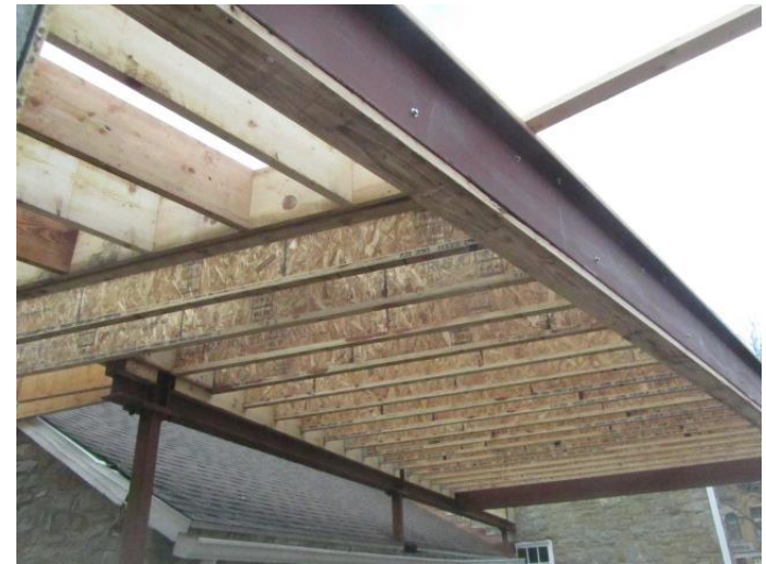
Flat roof framing over the circulation counter
