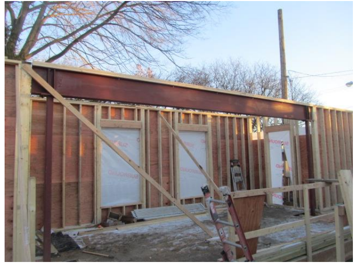
The final steel beam is placed at the children's room
