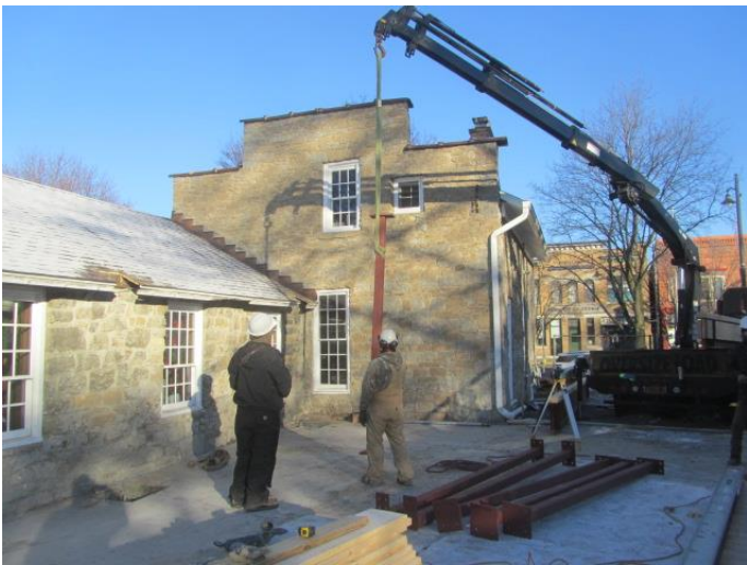
Setting the 1 st column
