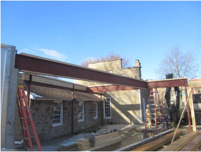
Beam 3 is connected to the 2 nd beam and elevator
