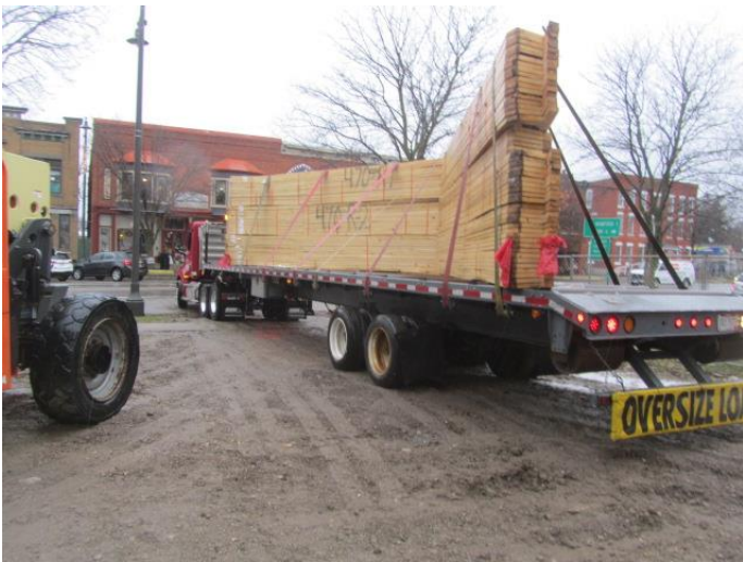
We received the roof trusses
