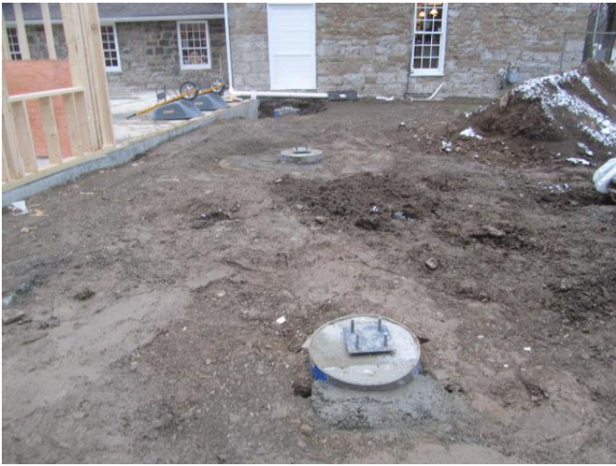
Overview of the piers
