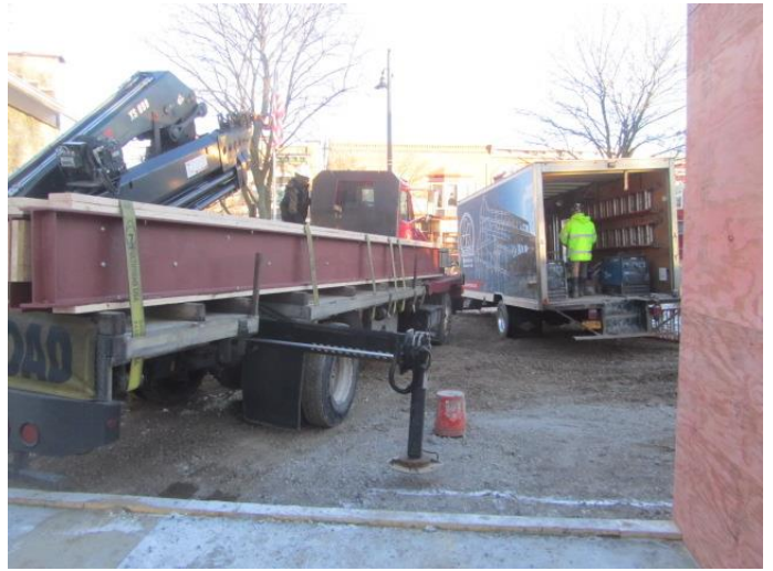
Kozel Steel is onsite with roof support beams
