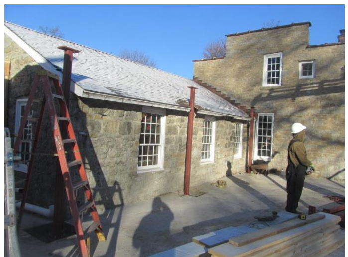
The 3 columns are set, ready for the 1 st beam
