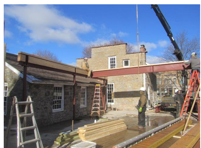
Setting the 2 nd beam
