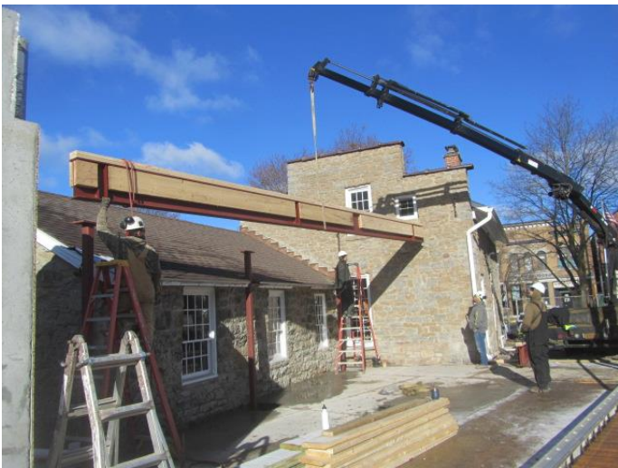
Setting the 1 st beam in place
