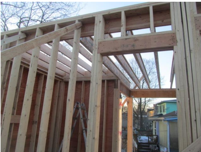
Flat roof framing over the bathroom
